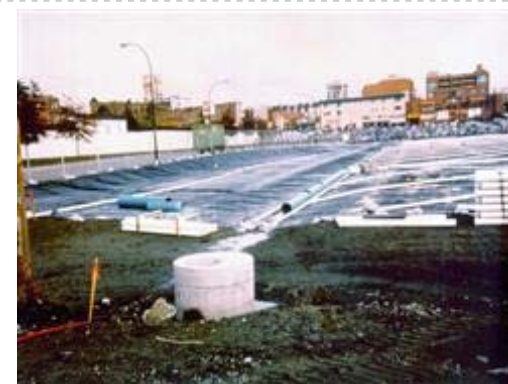
A GeoMembrane Cap in Vancouver, BC
