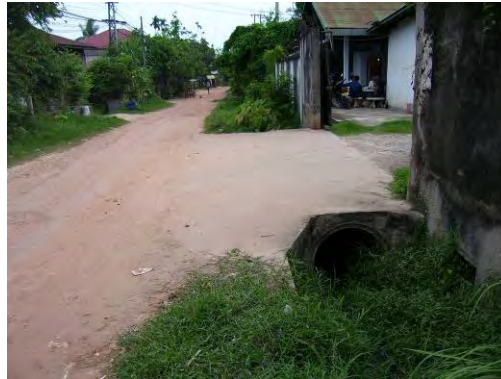
Lane immediately behind SPL site showing ditch which carries surface water from the SPL site.
